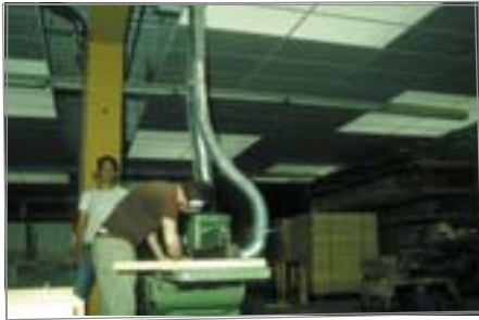
Figure 1: Sound-absorbent suspended ceiling in the carpentry workshop
